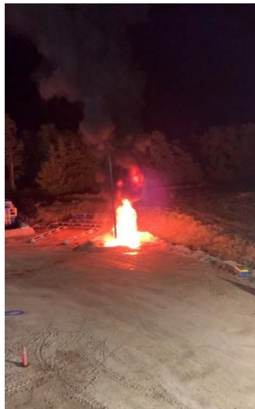
Figure 1—Fluid Overflow at flare.
