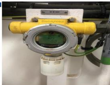
H2S Detector at Shale Shaker
