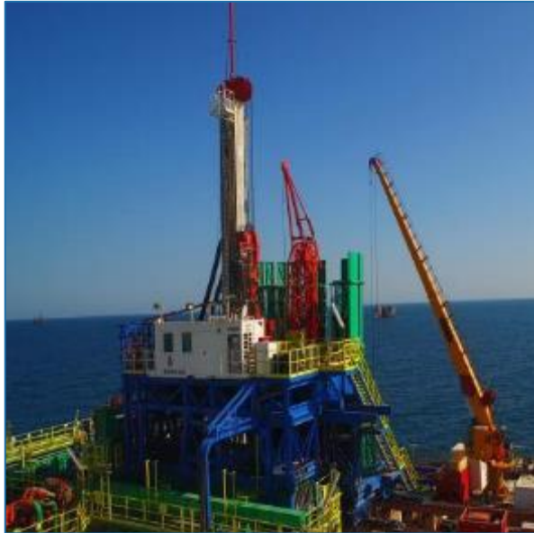
West Absheron Field Platform 20 (DRILLMEC HH300)
