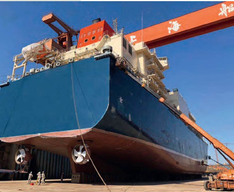
Construction of an LNG bunkering vessel in Shanghai.
