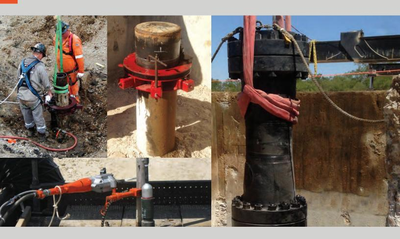
Our well control experts provide a range of options for wellhead removal services. Our pneumatic casing cutter and hydraulic sand cutter have the ability to cut various sizes of tubing and casing under pressure. The hydraulic nut splitter enables the removal of rusted, immobile studs. The hydraulic flange spreader removes seized flanges.
