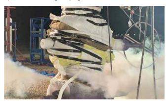
Crews freezed the frac valve below the flow tee, allowing us to test the plug while providing isolation from the well pressure. We rigged up a specialized freeze hose across the frac valve and connected it to a nitrogen transport. Once the hoses were rigged up, we pumped bentonite gel and nitrogen through the freeze hose, closely monitoring the temperature of the nitrogen during the entire freeze operation.
