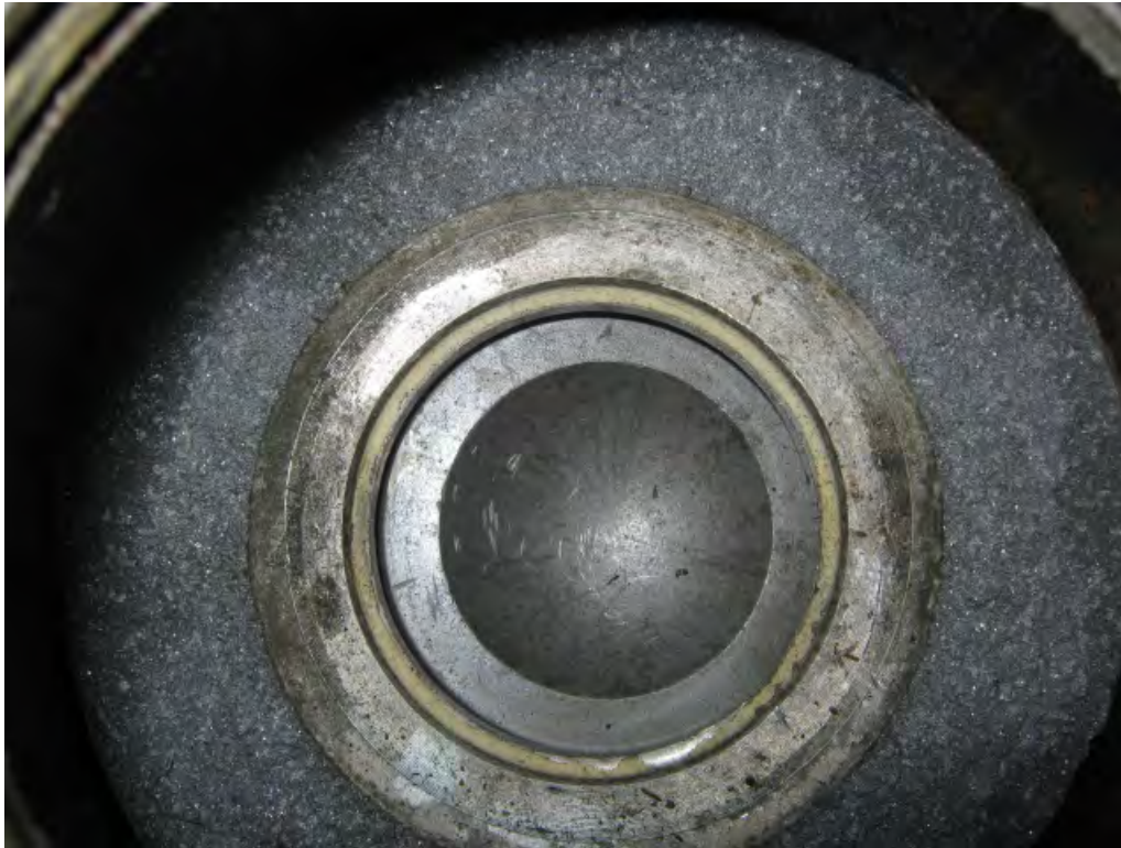
Figure 3.19: Close-up Photograph of Flapper Assembly Failure
