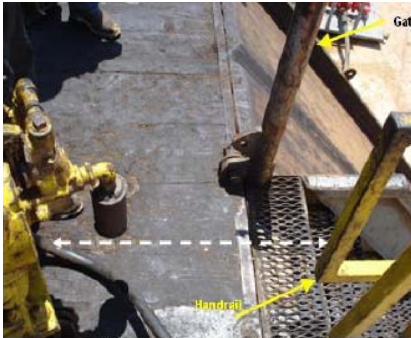
Air hoist and hand rail after installation
