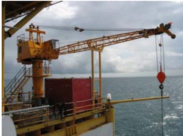
Crane before incident
