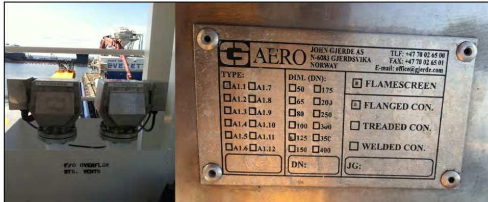
Photo 4 - Fuel Oil Overflow Vent (Typical)
