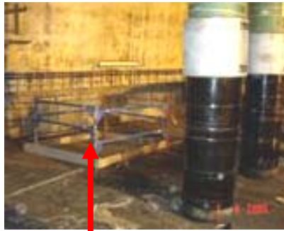
Barriers around the manhole after the incident with general lighting on
