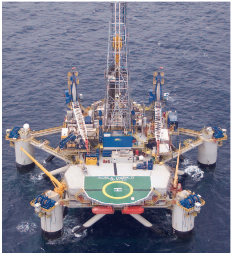
The semisubmersible Noble Therald Martin is one of the company's rigs that is contributing to Noble's efforts to reduce its emissions profile.
