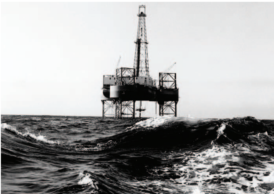
LeTourneau's first jackup, Scorpion built for Zapata Offshore, on location in the Gulf of Mexico. The rig was built in 1955 in Vicksburg, Miss, and "walked" to the Mississippi River under its own power.
