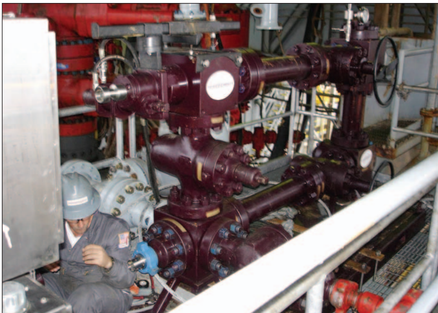
Figure 5: Installing the flow choke manifold section of the closed-loop MPD system.
