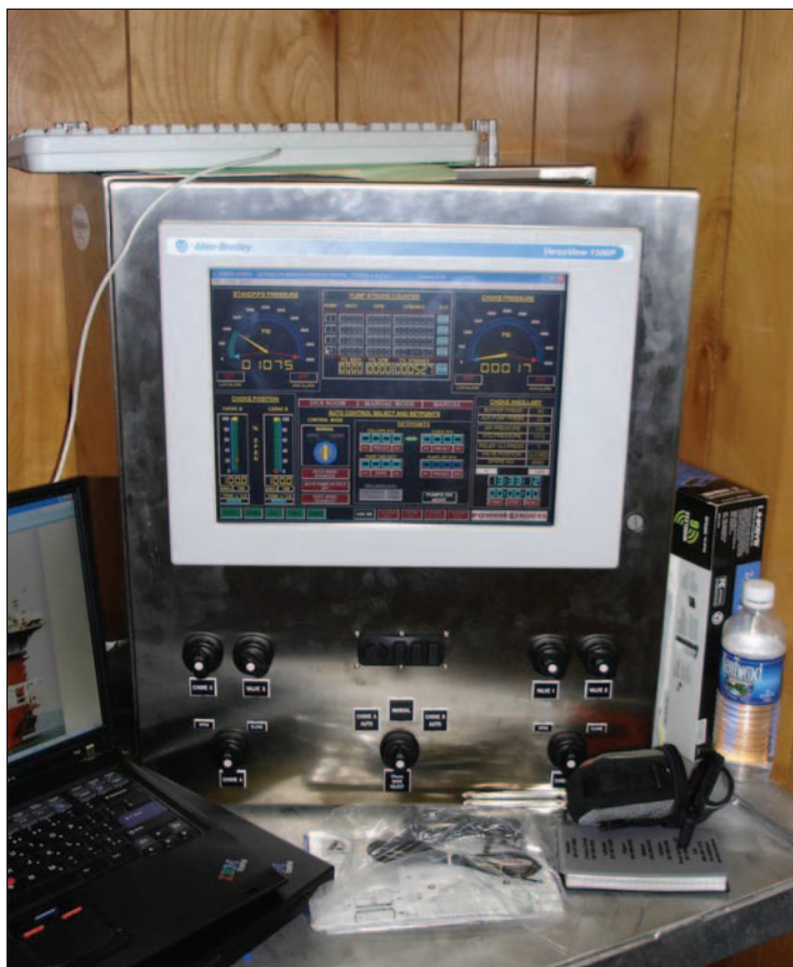
Figure 3: The Automated Managed Pressure System continually receives new pressure updates from the well model and then automatically modulates the choke to achieve the desired annular pressure. The Main Operating Screen is shown here.
