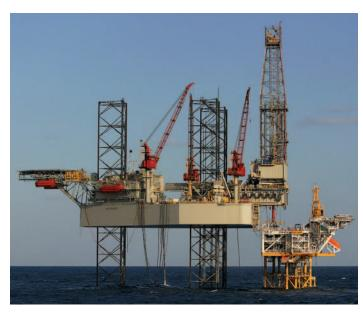
Keppel FELS is building two KFELS 'B' Class jackup rig for Awilco similar to the one pictured above. The rigs are rated to drill in up to 400 ft of water. Delivery is scheudled January 2007 and January 2008. Photograph courtesy of Keppel FELS.
