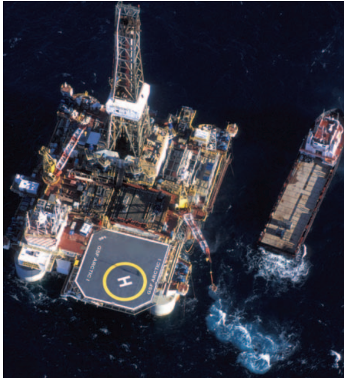
GlobalSantaFe's semisubmersible GSF Arctic I was drilling in the US Gulf of Mexico before mobilizing to Venezuela last year. The contractor's fleet is covered under the maritime security regulations developed by the US Coast Guard as a result of 9/11.
