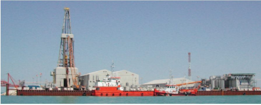
KCA DEUTAG's T-47 rig operates from an artificial island in the Caspian Sea. The rig was recently modified to enable it to skid over all seven existing well slots.
